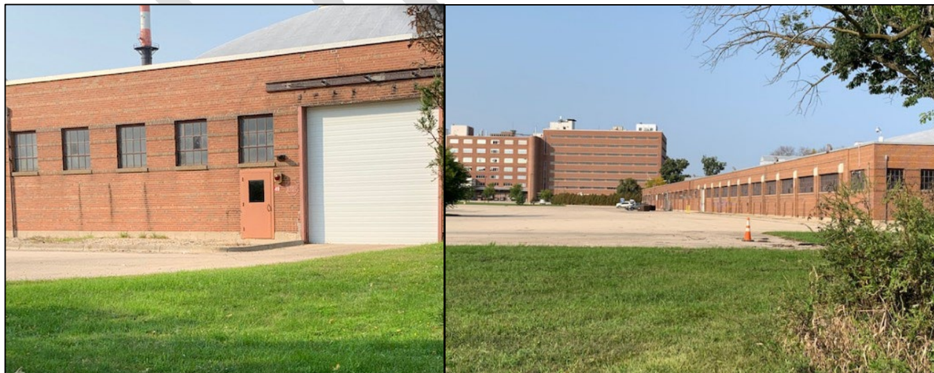
Figure 8. The south side of the Bodgery building adjacent to the former 1,2-DCA tank site
