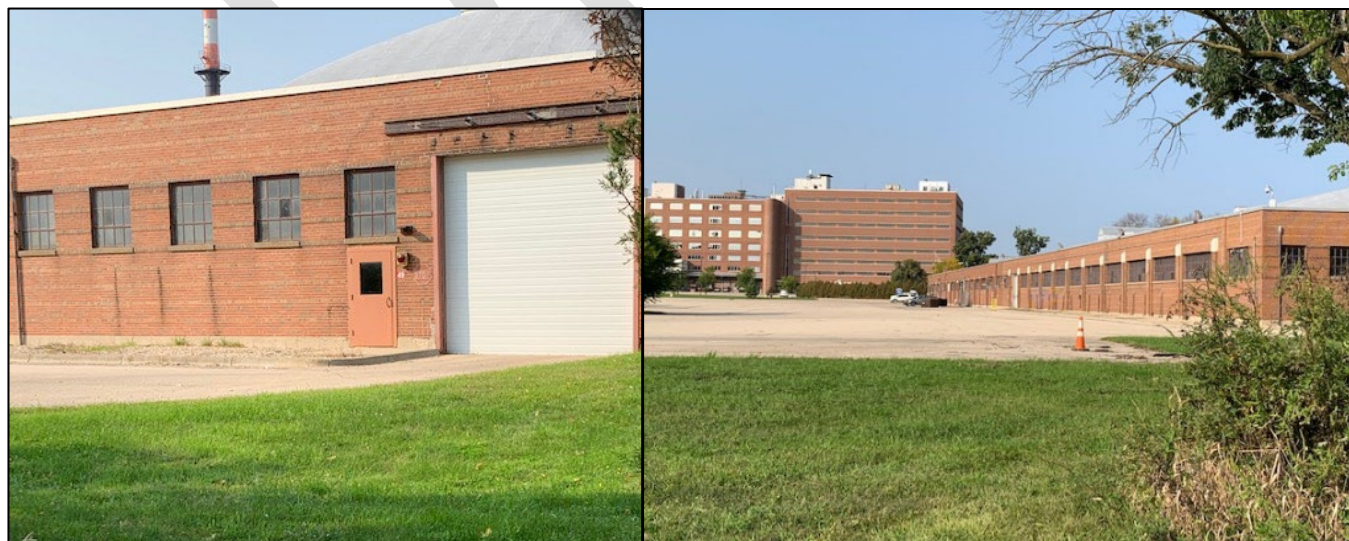
Figure 8. The south side of the Bodgery building adjacent to the former 1,2-DCA tank site
