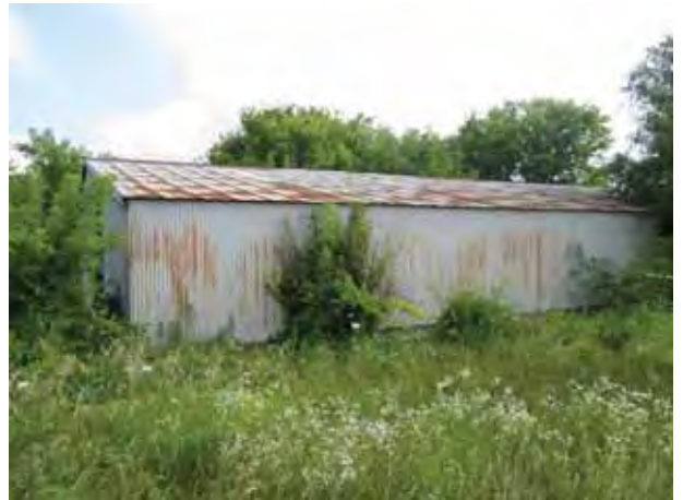
Photo #10 South Side of On-Site Building
