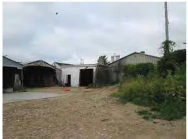
Photo #18 Vacant Buildings to the West
