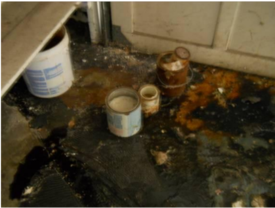
Material behind salt pile in loading dock area.
