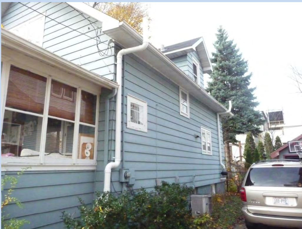
Showing two separate depressurization systems on the north side of this home on Marquette Street. Note the location of the 2 vapor depressurization systems relative to the 2 rain gutter downspouts.
