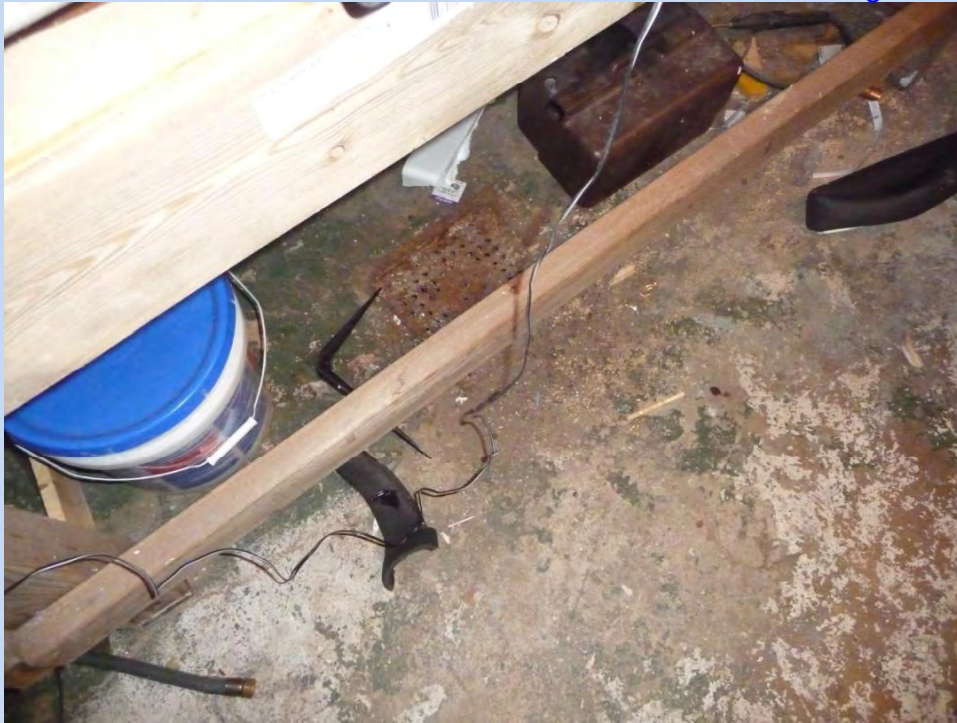
Shows the presence of floor drains in the basements which would act as conduits for vapor to enter the buildings.
