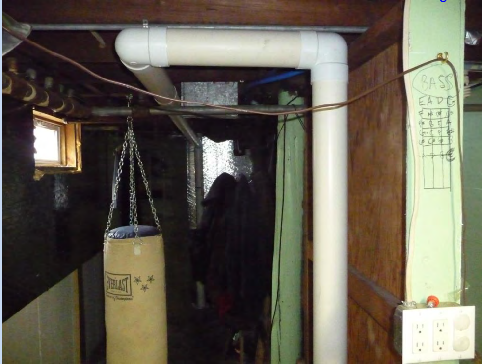
Showing how the two vapor extraction locations are plumbed together to the outside.
