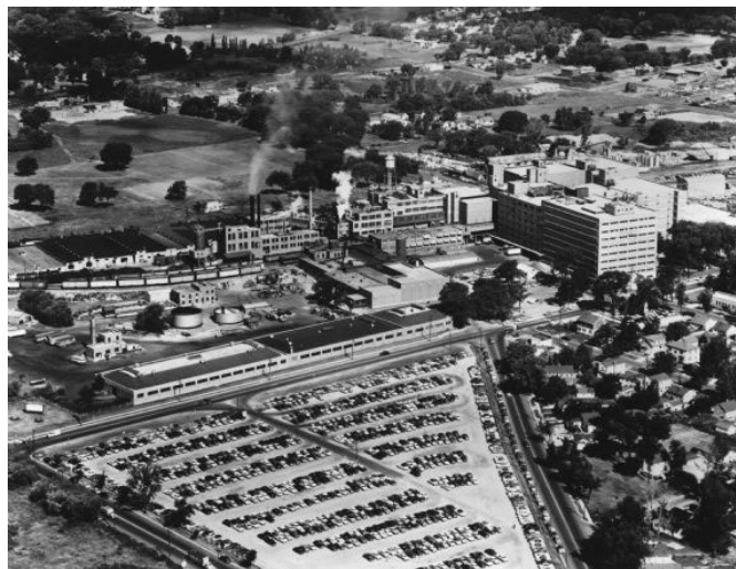
FIGURE 5: Street Grid Pre-Packers Avenue Construction
