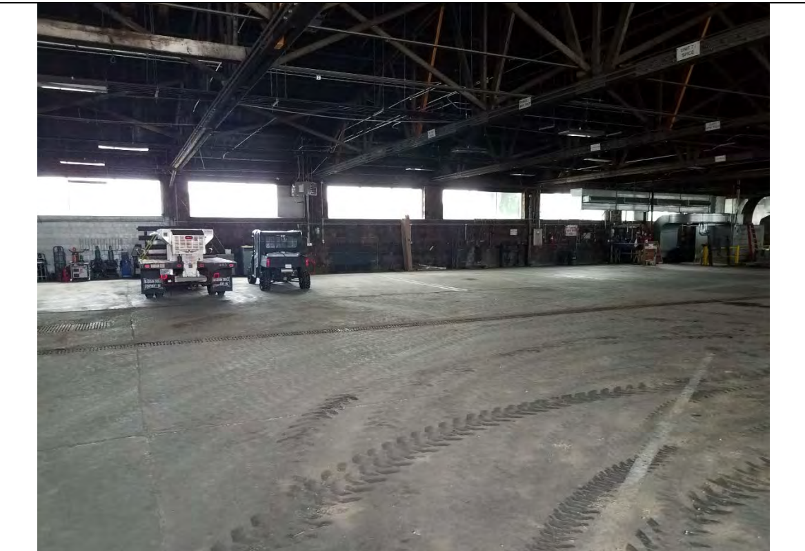
Photograph: 20 Interior of portion of Building 20 used for storage
