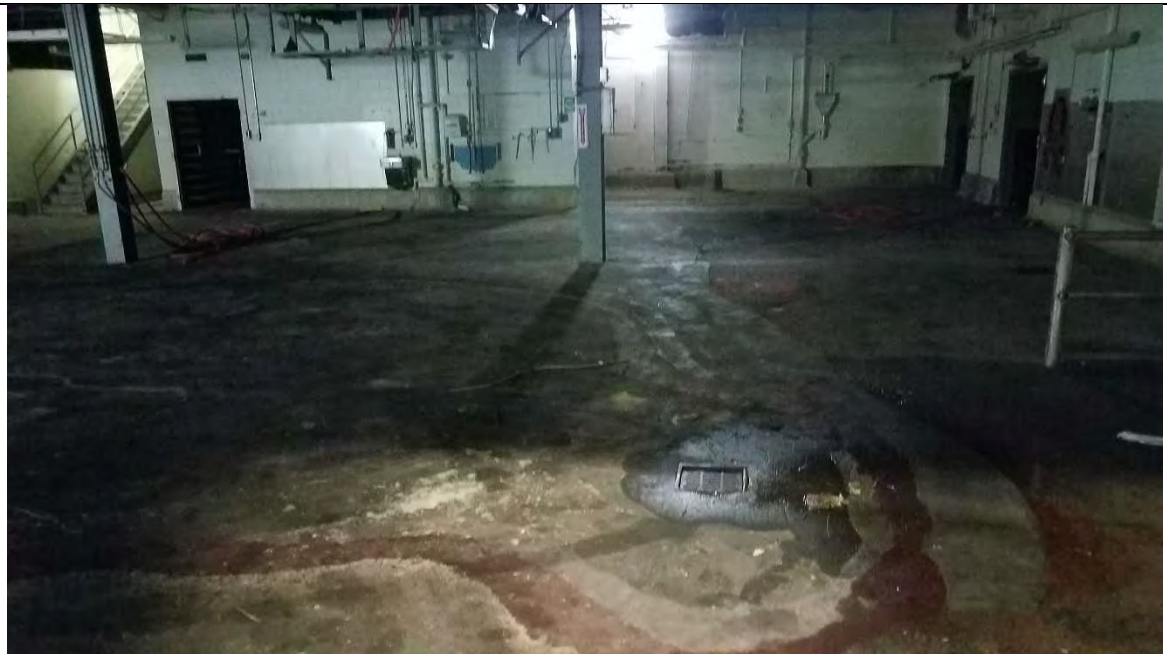
Photograph: 9 | Sub-slab vapor pin location in vicinity of former Spice Room
