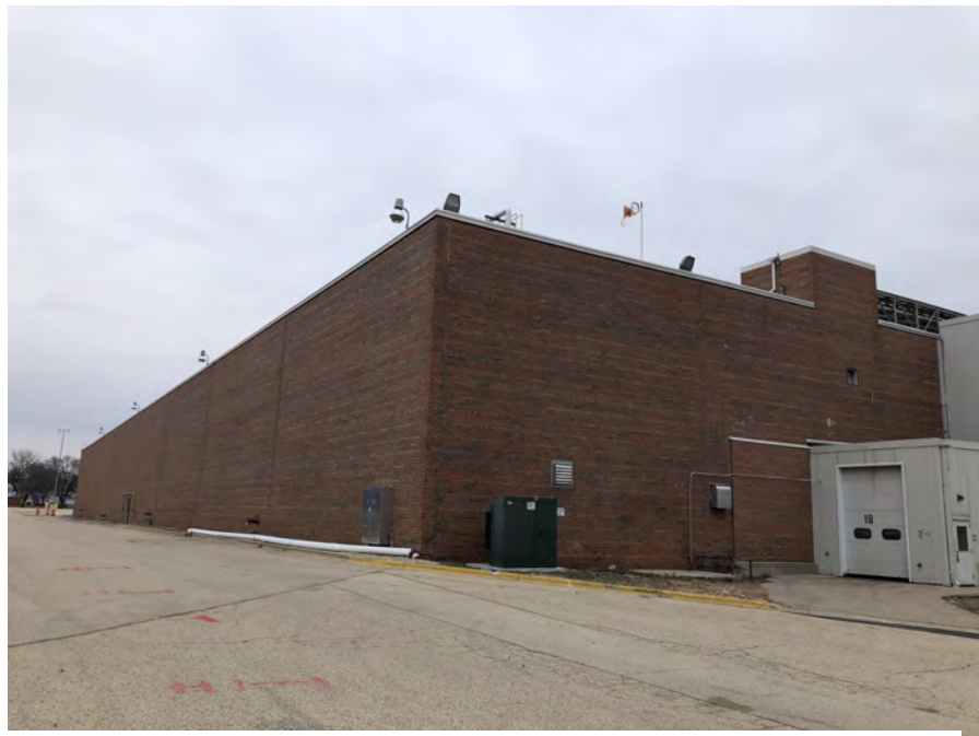
Photo 2: View of building 43 from the southwest.
