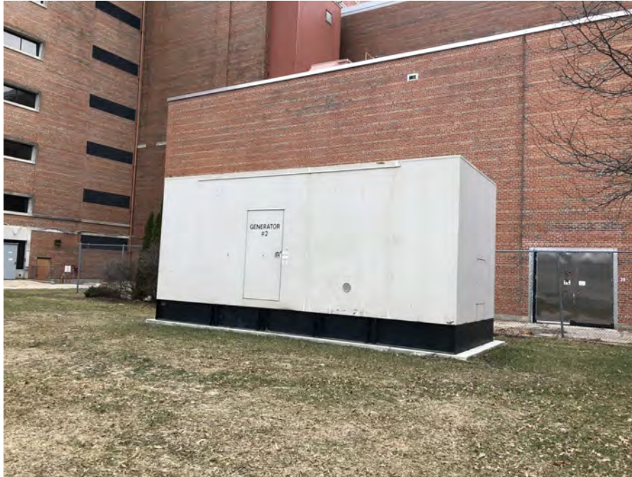
Photo 7: View of the emergency generator form the east.
