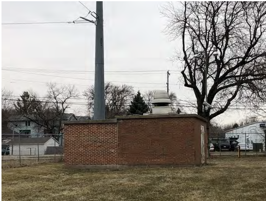
Photo 4: View of the Wellhouse from the south.
