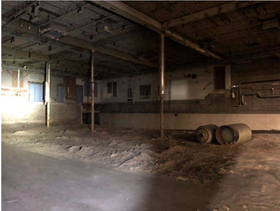
Photo 11: View of the former mezzanine in Building 50.
