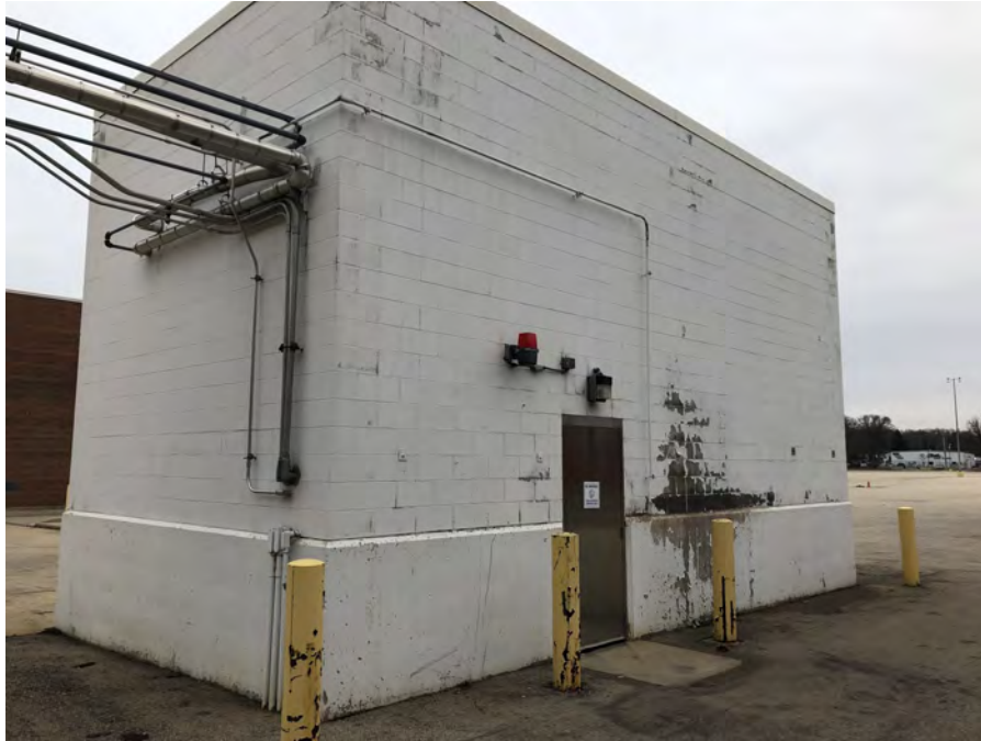
Photo 3: View of the Brine Building from the southeast.
