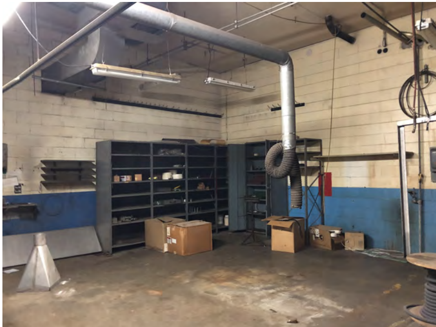
Photo 8: View of the former weld shop in Building 43.
