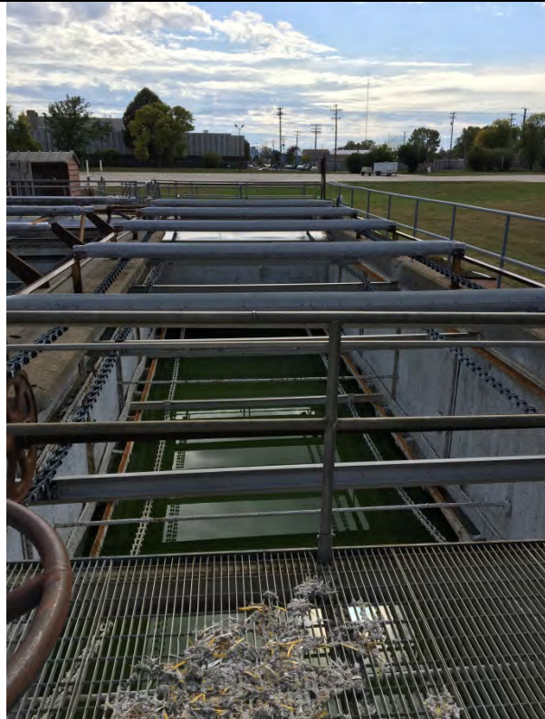
Photograph: 6 Skimming pond of the non-operating on-Site water treatment plant.
