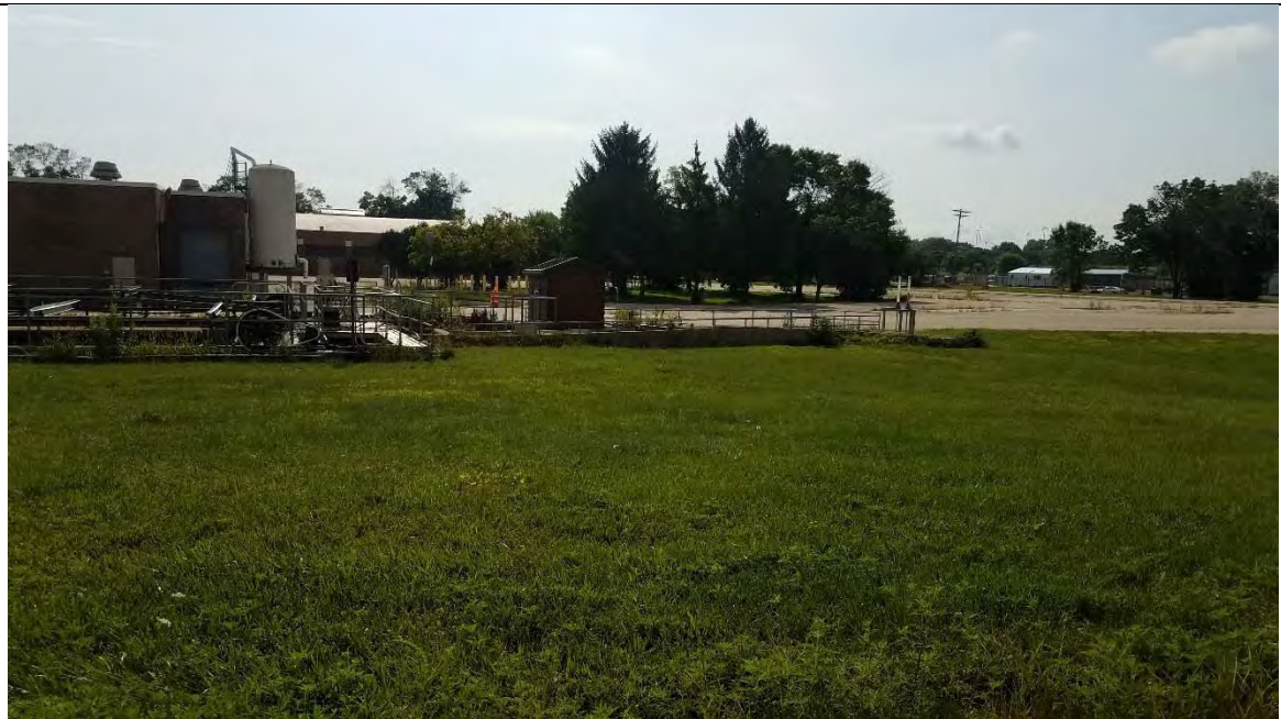
Photograph: 7 | Monitoring wells installed in vicinity of former Ethylene Dichloride ASTs
