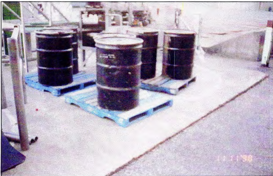
Photograph 4 Six drums of soil and water removed from casing using vacuum truck.
