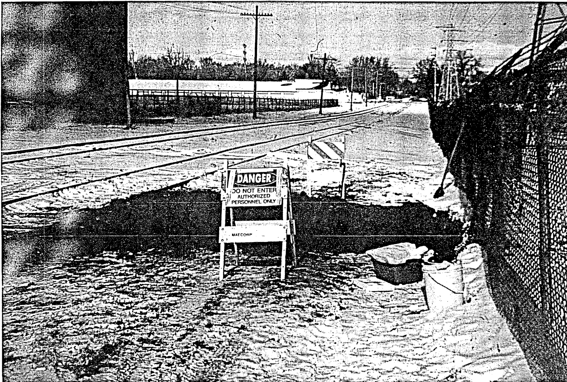
AREA B-5 EXCAVATION
