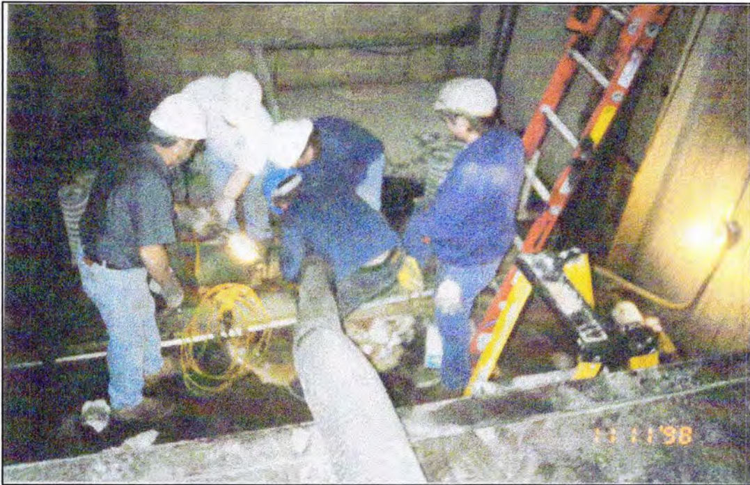
Photograph 3 Evacuation of from casing using vacuum truck hose.
