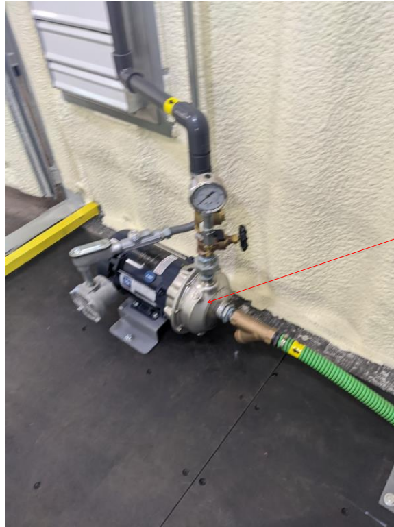
Figure 7: Transfer Pump and Knockout Water Sample Port
