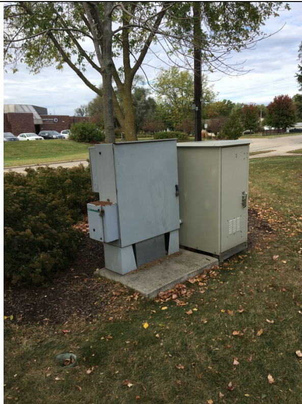
Photograph: 6 ERM observed one transformer at the site. The transformer appeared to be in good condition and the concrete pad was not stained or damaged.
