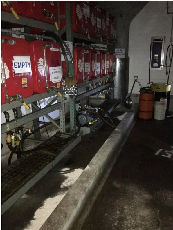
**Photograph: 11** Former oil storage area in the basement of the facility. A rack of oil containers remained in place, but all level indicators appeared to be empty.
