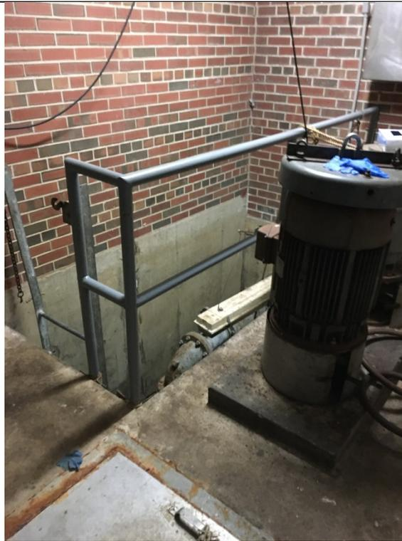
**Photograph: 15** Sump room on ground floor historically tied into the on-Site water treatment plant. This particular sump was not currently collecting water, though the pump remained powered on.
