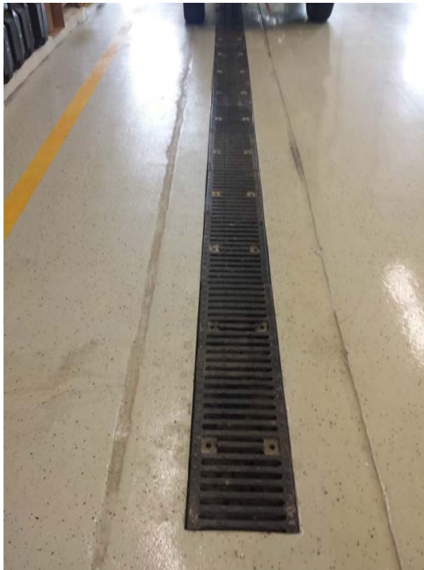
Photo 2: Trench drain (one of several) in the Fire Station (Building 430)
