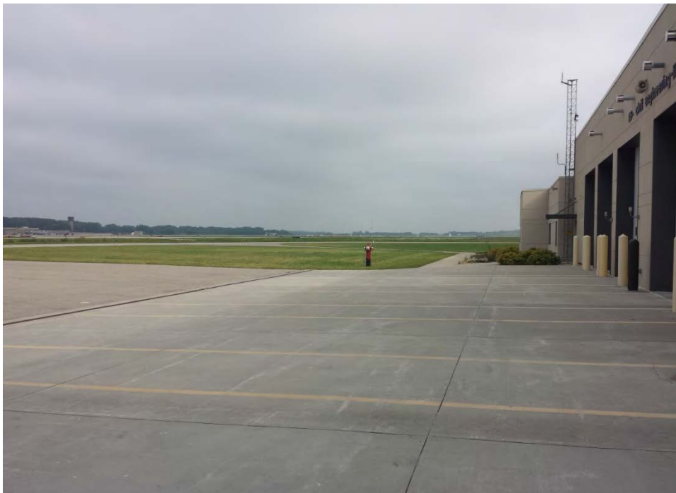
Photo 4: Looking north on west side of Fire Station (Building 430) where vehicle spray pattern tests are conducted.
