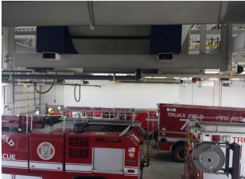
Photo 1: Overhead foam fill at Fire Station (Building 430).
