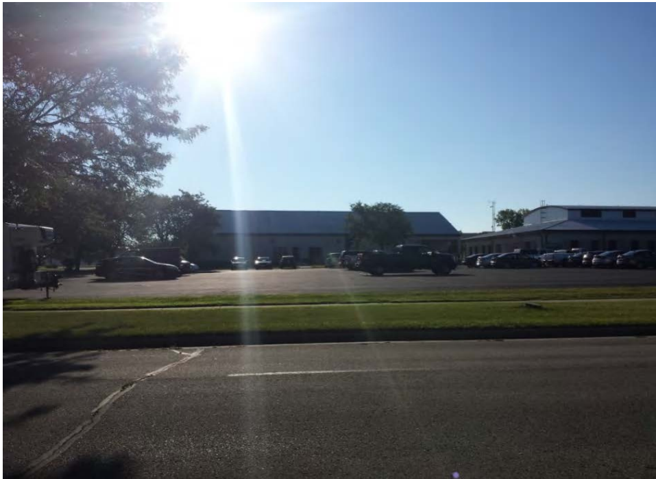
Photo 11: Looking east toward parking lot west of Building 503 where soil from 1981 fuel spill was placed on top of concrete pads and later disposed offsite.
